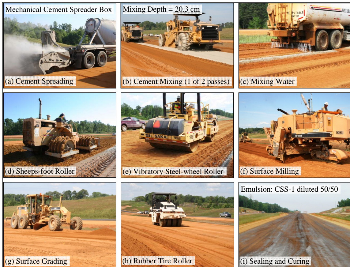
Figure 1.1 Soil-Cement Base Course Construction on State Route 9 (April 2012)
