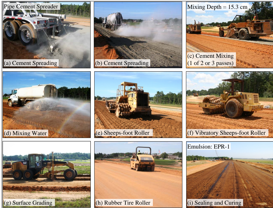
Figure 1.2 Soil-Cement Base Course Construction on State Route 475 (June 2012)
